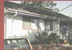
Cladding hiding fibro walls
